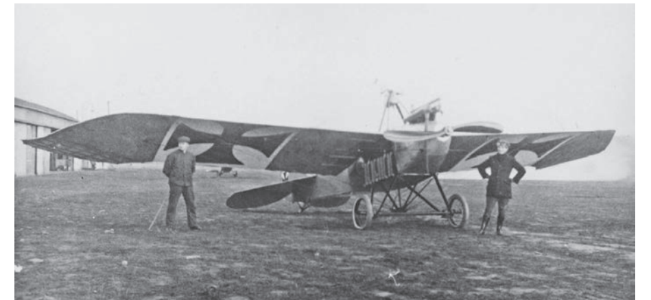
Perhaps one of the most recognizable aircraft to appear early in the war, the Austro-Hungarian designed Taube was built by at least 14 companies with a great many variations on the initial design. It proved to be unsuitable for front-line service and was relegated to use in training of new pilots.
